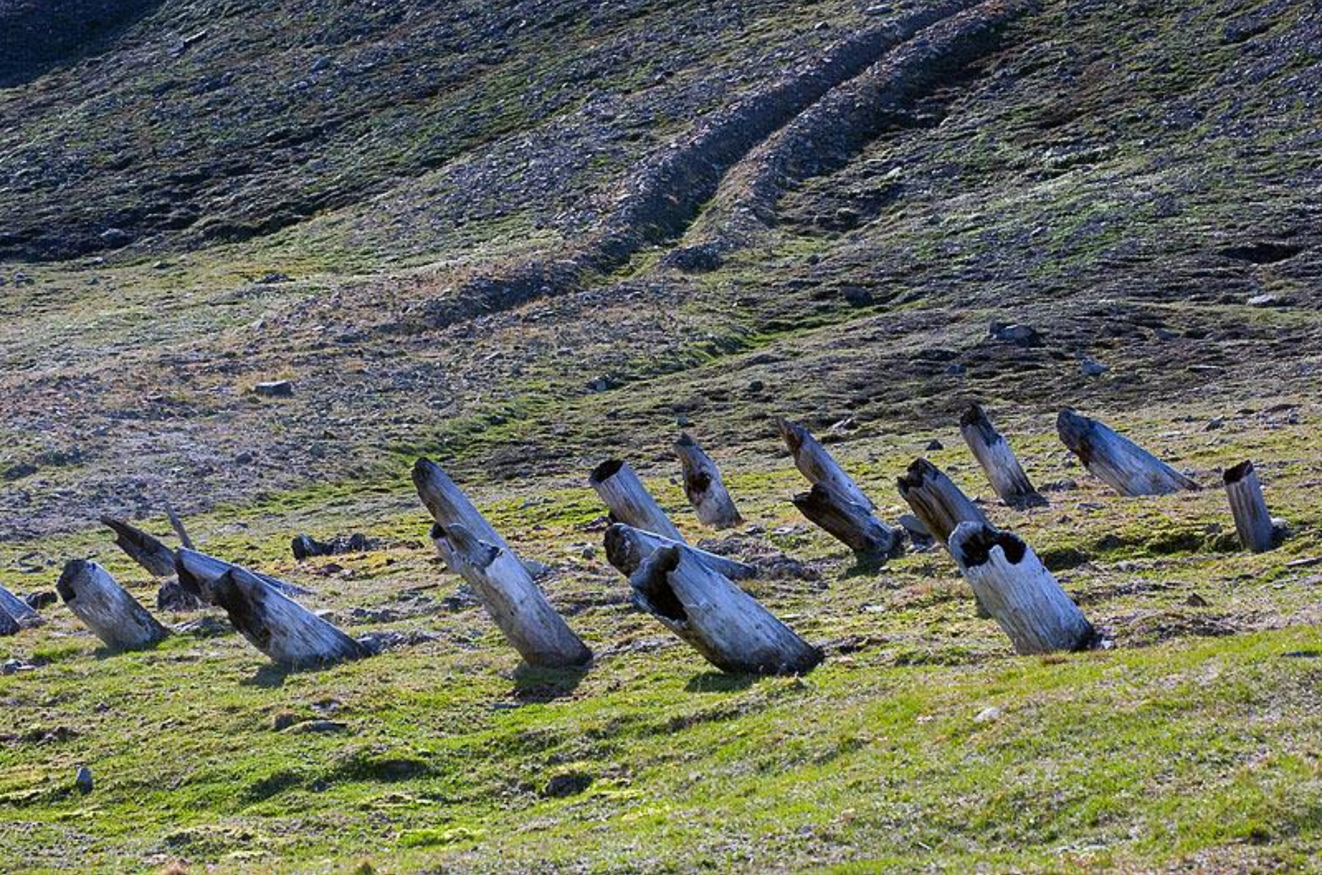
Solifluction is evident in Longyerbyen where posts formerly used as foundations of tramway pylons have tilted downslope (JA)
