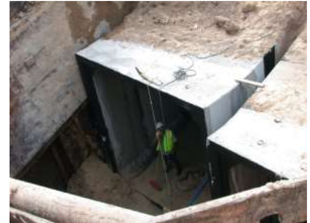
The installation of large new culverts under Kirby, Cambridge, & Hermann
