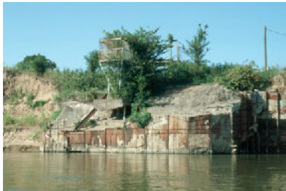
Figure 10. Pump station near Kirtley. Water from the Colorado is still pumped for stock and crop irrigation.
