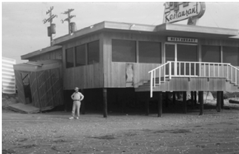
Restaurant on the Gulf Beach at Port Aransas after Hurricane Carla, September 1961, showing removal of the sand from under the restaurant. Pictured is Walter Siler, who was a student at that time. Photo provided by Ernest L. Lundelius.
