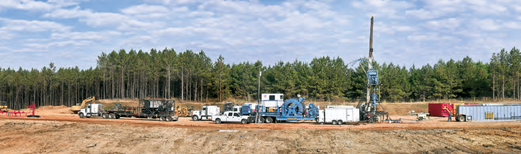
Work progresses at a $34 million Department of Energy funded research project evaluating sequestration and monitoring strategies for long-term storage of carbon dioxide at Cranfield field in Mississippi. Here, an observation well is being drilled and fiber-glass casing is waiting to be inserted and cemented inside the well.
