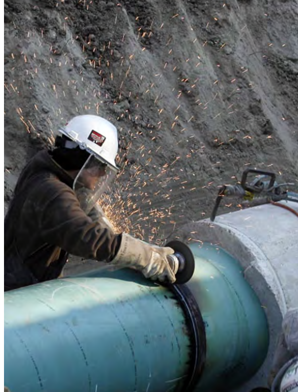
Contractor works on a joint of the 24-inch carbon dioxide pipeline that will stretch more than 300 miles from near Donaldsonville to Houston. U.S. Source: Baton Rouge Advocate.
